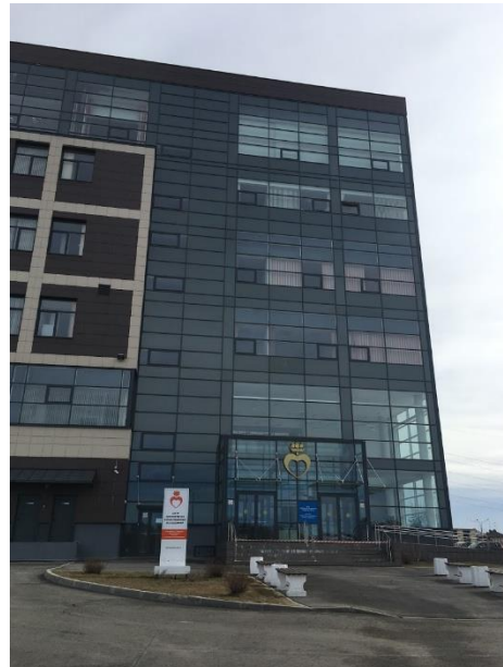
Picture 2 The building where I researched
